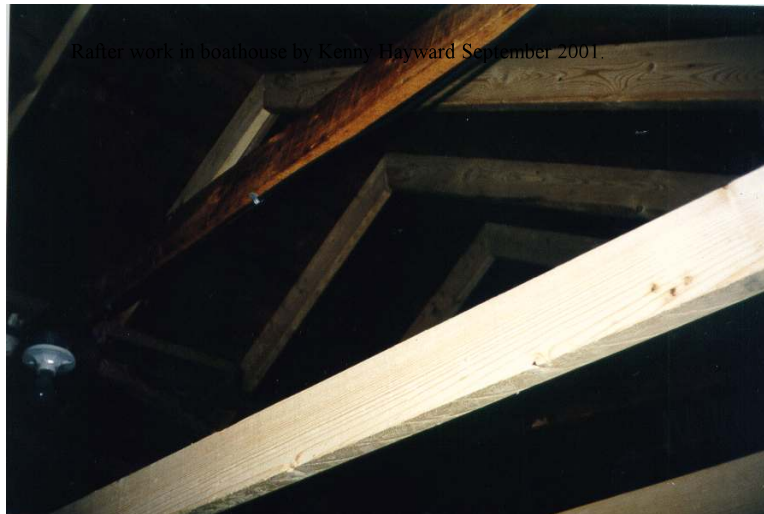
Rafter work in boathouse by Kenny Hayward Sept. 2001.
