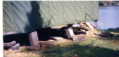
Poor drainage allowed trapped water to freeze and damage the footings.
