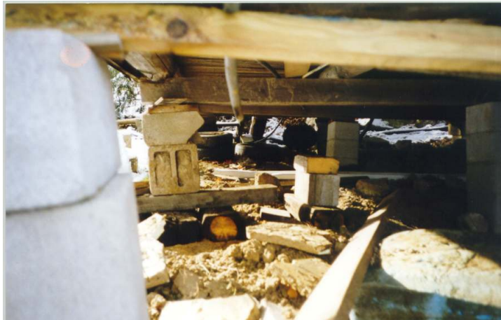
Fall 1997. Ongoing work on footings.
