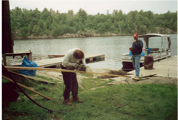
June 1994. Start of shower building.
