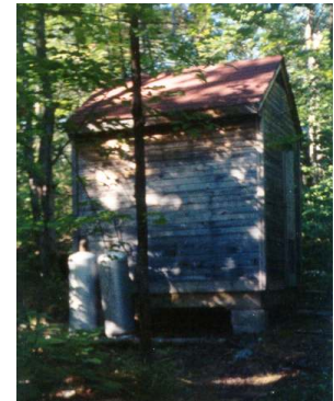
Shower building. Picture August 1999.
