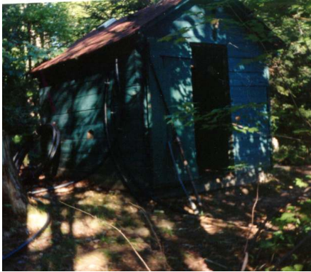
Power plant building.
