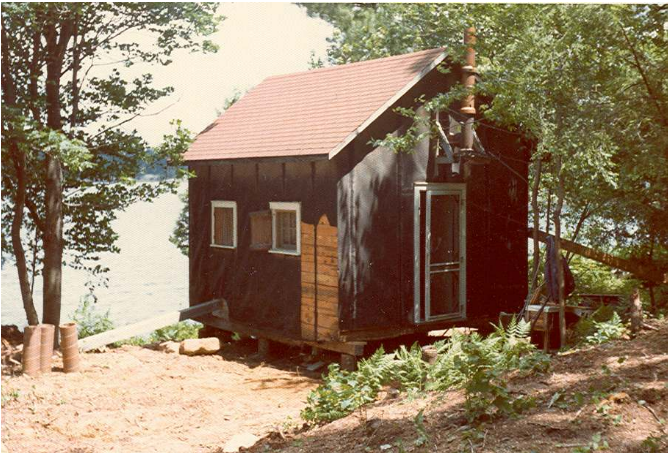
Original Cook's Cabin
