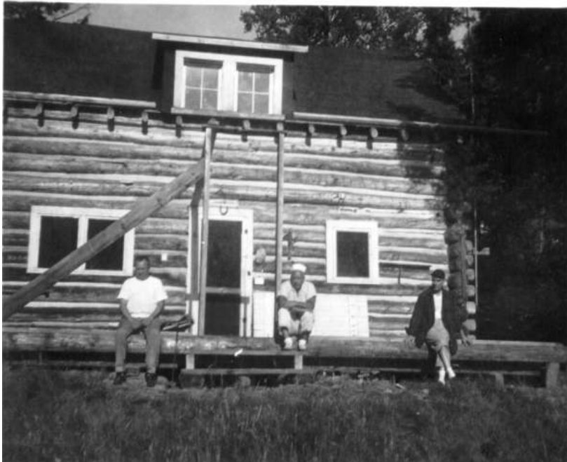
Old porch removed and framing of new porch started.
