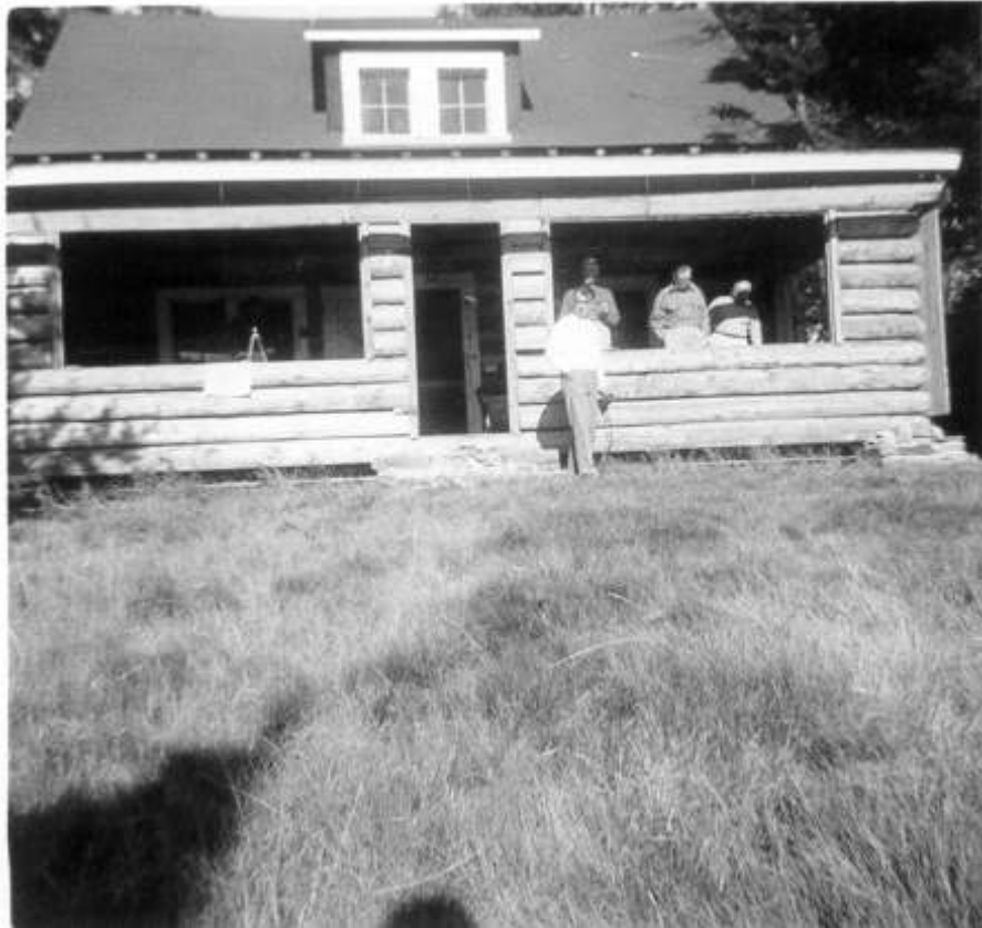
Final stages of construction.
