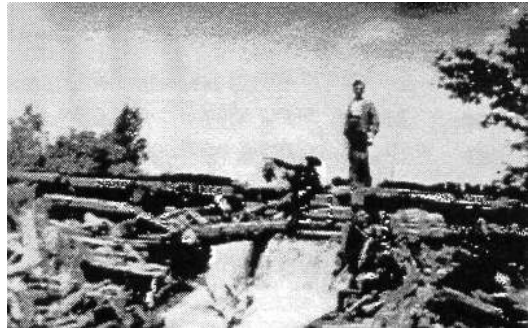
Farm Creek logging chute 1943.
