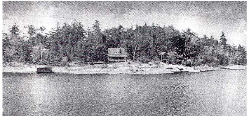
Morton's Point Camp soon after the construction of the dormer in 1937.
